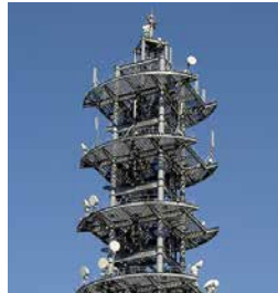
Large-zone base station that secures communications in densely populated areas in times of disaster
